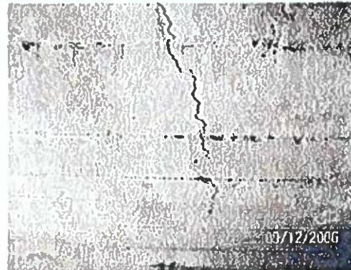
Figure 27 and Figure 28 – Cracked Concrete Box Culvert / Bridge
