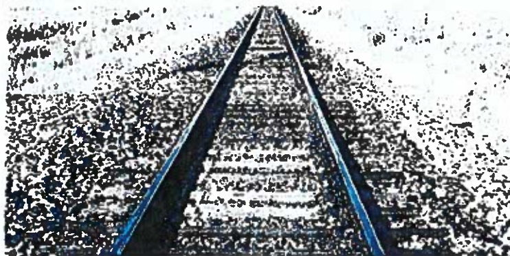
Figure 16 – Good Cross Section on the UPRR Main Line
