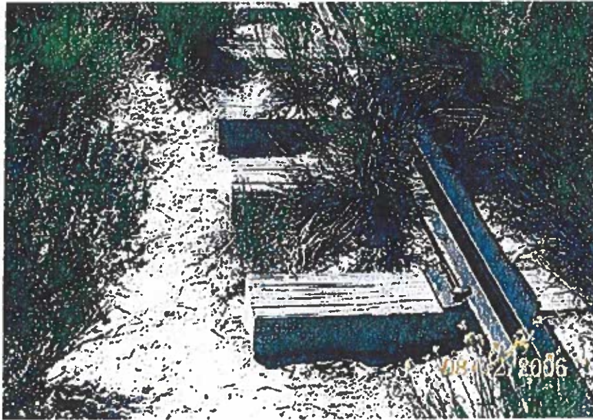
Photo No. 9 Mile Post 40.4, Exposed Ties at Edge of Siding
