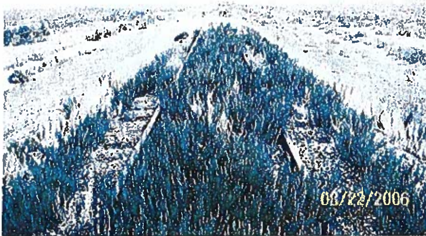
Photo No. 4 Mile Post 52, Looking South, Typical Side Swales Indicating Borrow Areas Adjacent to Embankment
