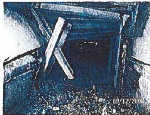
Figure 22 – Collapsed Wood Culvert
