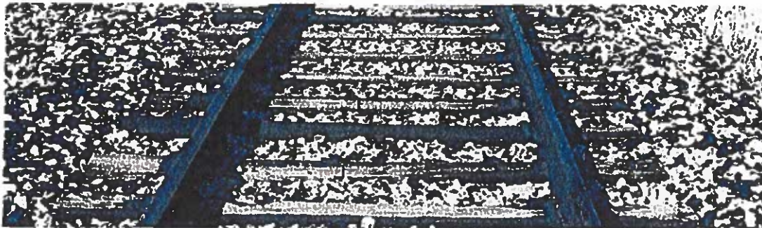
Figure 4 – Example of Relatively New, Good Quality Ties on the UPRR Main Line
