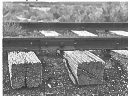
Image 1: This site survey photo shows poor tie condition represented in some portions of the line.
