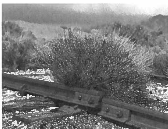
Figure 2: A broken joint bar on the 60-pound mainline rail near Cherry Creek (MP 91.3) is indicative of the condition of the NNRV Mainline.
