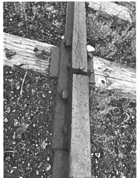
Image 2: This site survey photo shows general state of rail and joints along the entire line – note head cracking.
