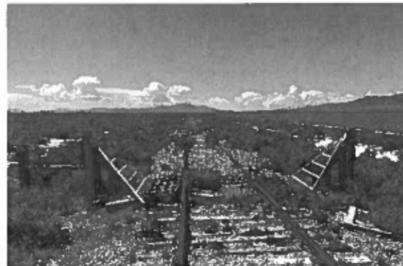
Figure 5: One of 22 cattle guards / fence crossings along the NNRV main line, each of which will be replaced / upgraded.
