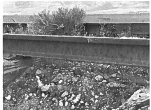
Image 4: This site survey photo shows the general state of ROW roadbed, including ballast section loss.
