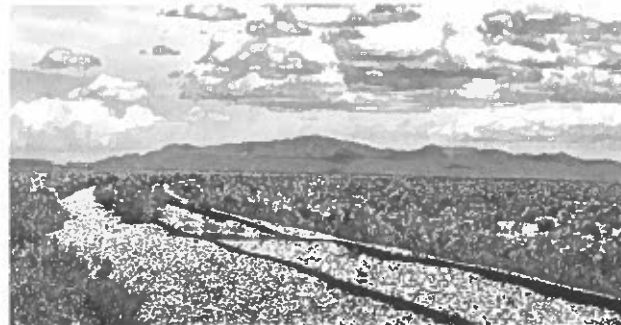
Figure 5: The mainline at MP 87, as photographed in May 2023. Note the poor surface of the railroad and washed-stone ballast.
