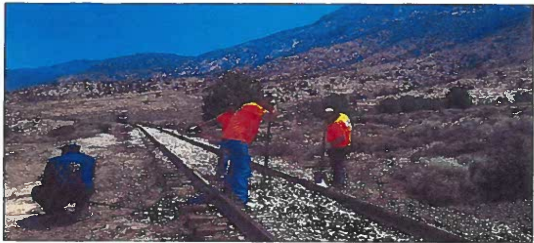
Tamping the ballast in place, the kink is gone.
