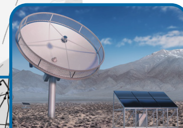
26' x 20' antennas and low-frequency dipoles powered by solar panels
